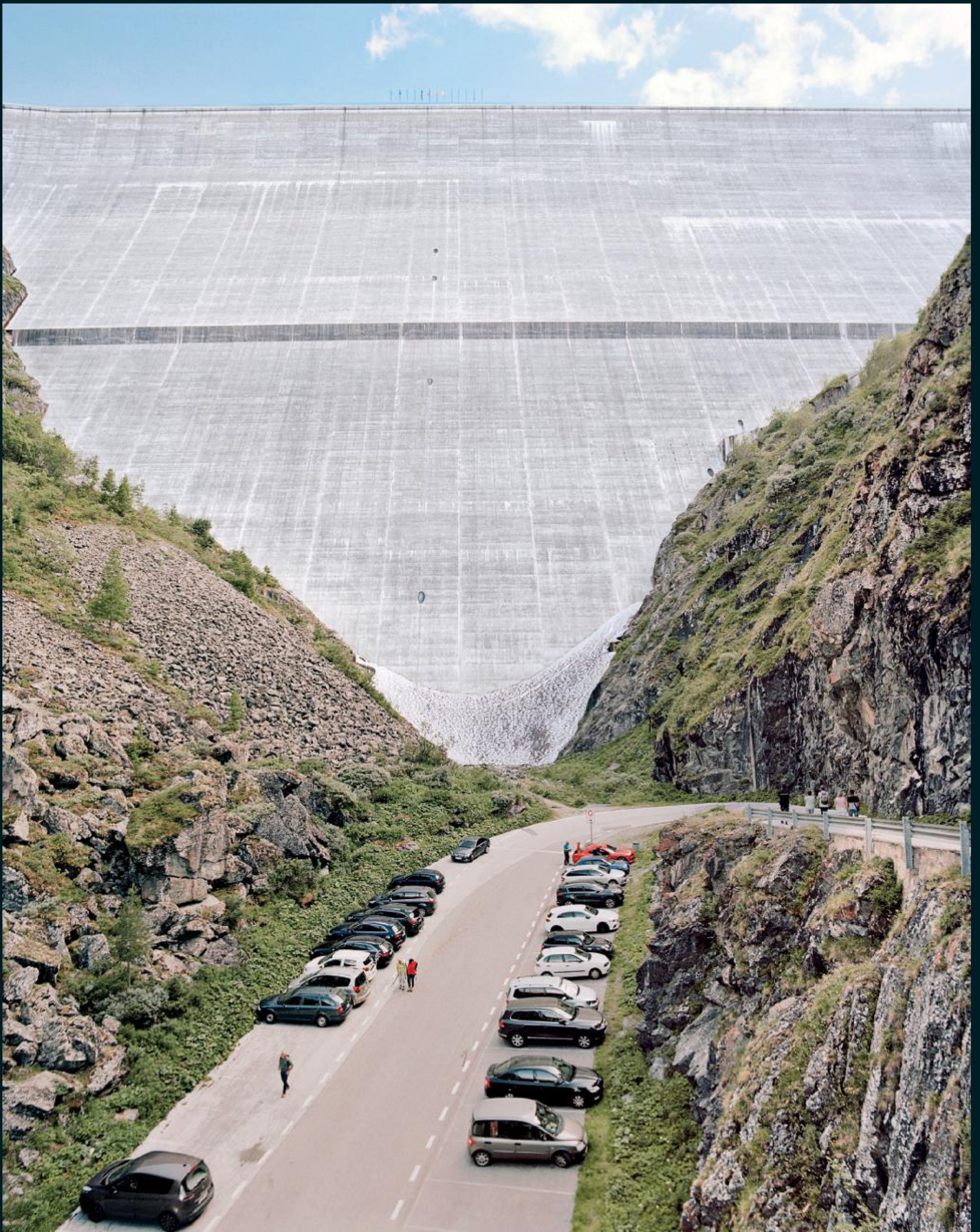
Grande Dixence, 935 feet high, is the world's tallest gravity dam. Built by 3,000 men in the middle of the last century, today it's part of a complex of dams and reservoirs that produces enough electricity to power about half a million homes.
