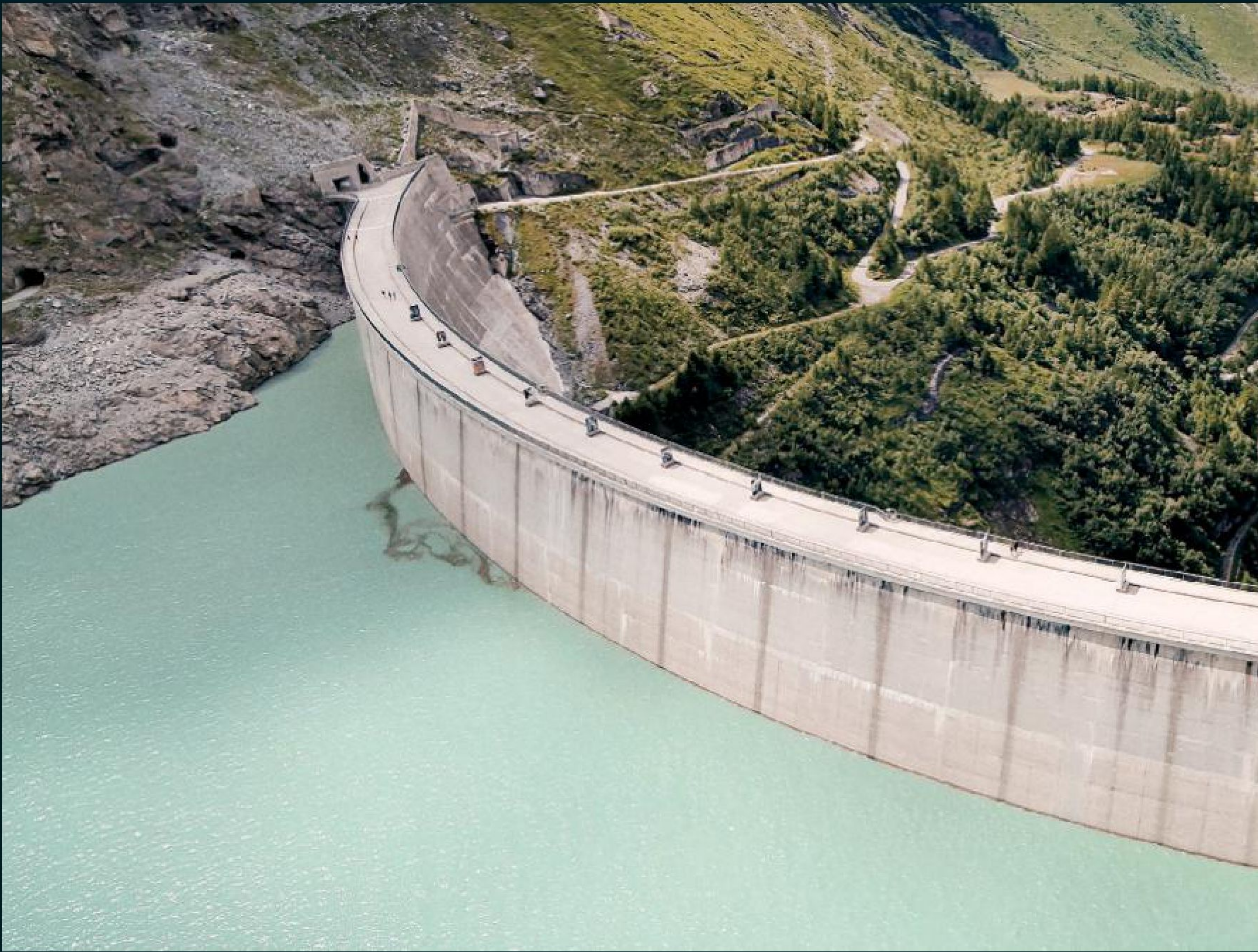
At 820 feet, Mauvoisin is the second-tallest dam in Switzerland and the biggest arch dam in Europe. (Arch dams curve inward toward the water they contain.) More than 1,800 workers built it over a decade, finishing in 1958. The tunnels they used are open to tourists today.
