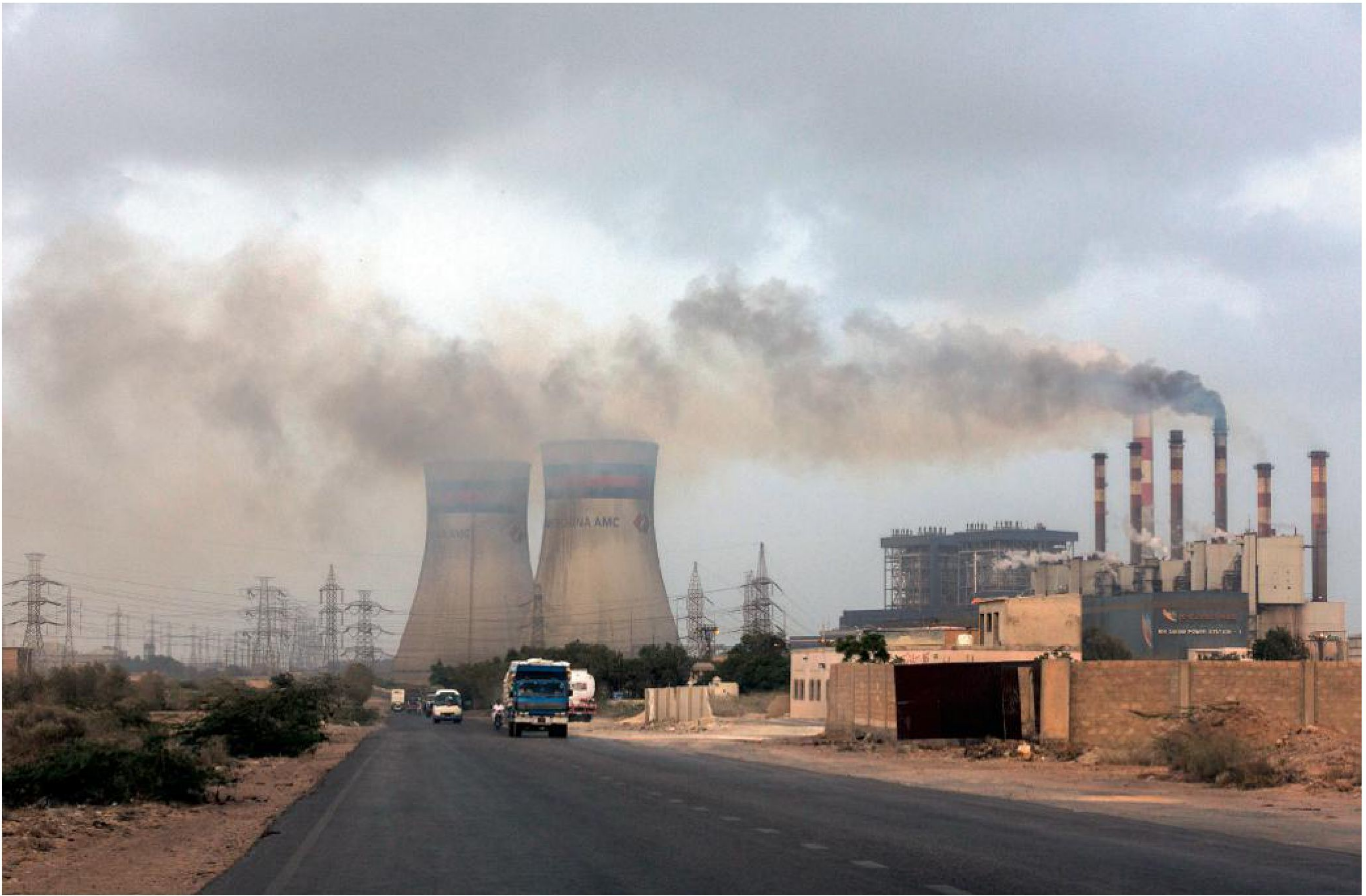
At Port Qasim, smoke from an older oil-fired power station (right) drifts across a newer plant that burns imported coal
